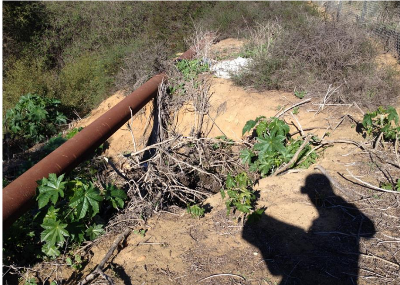
Photo 1: Severe erosion in southeast corner of open space boundary; photo taken looking north.
