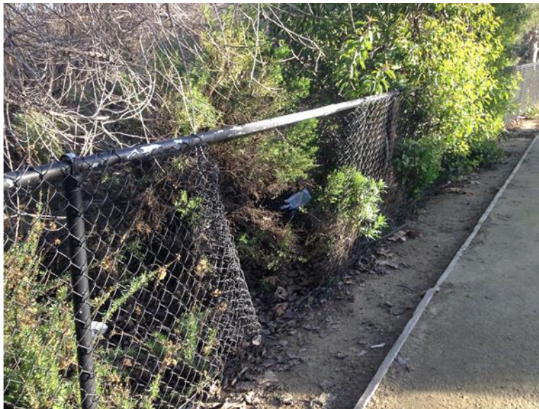
Photo 10: Tear in fence adjacent to parking lot on the western boundary of open space .
