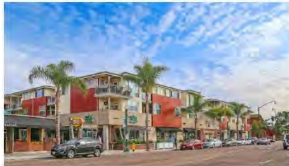
Figure 12: Pacific Station Development, Encinitas
