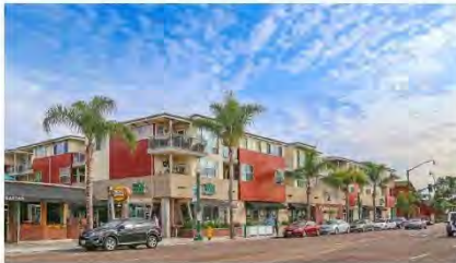
Figure 12: Pacific Station Development, Encinitas
