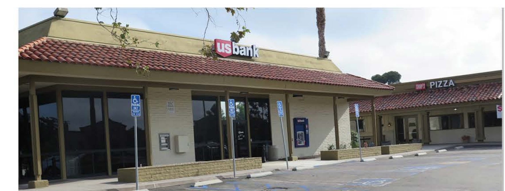
Big box stores are complemented with strip commercial stores such as banks, restaurants, and other retail services.
