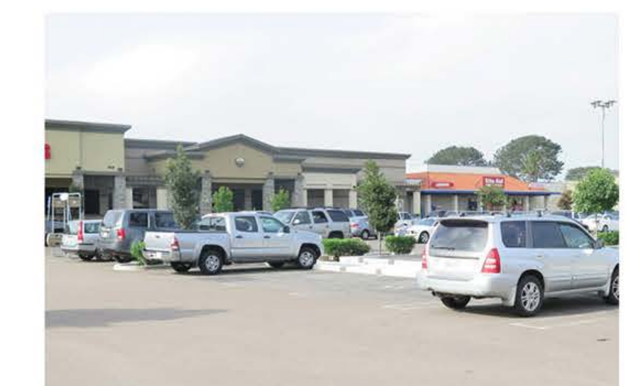
Large, surface parking lots are located in front of buildings.
