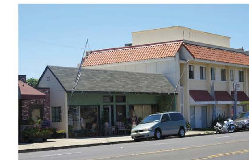
Development along the corridor tends to be a mix of one and two story structures which express individuality.
