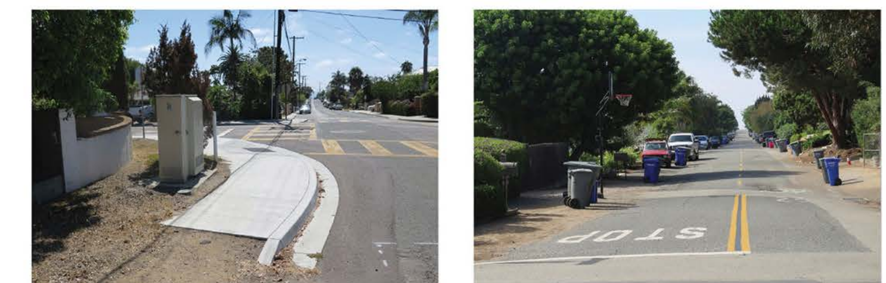
Some curbs and sidewalks have been added, but are not consistent.
