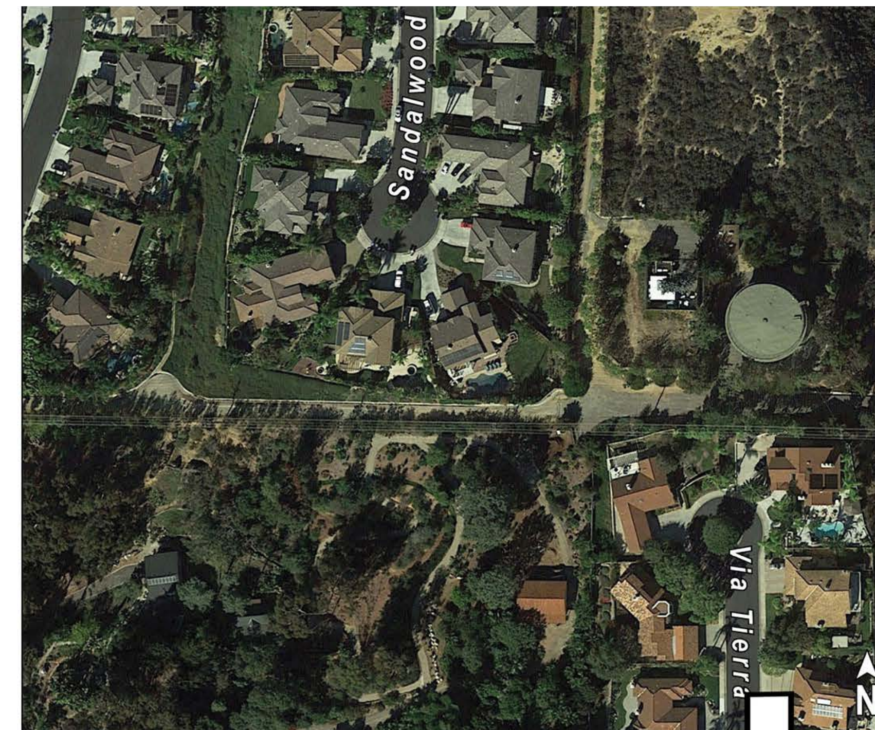
Snapshot Area #2 - Aerial Photograph
