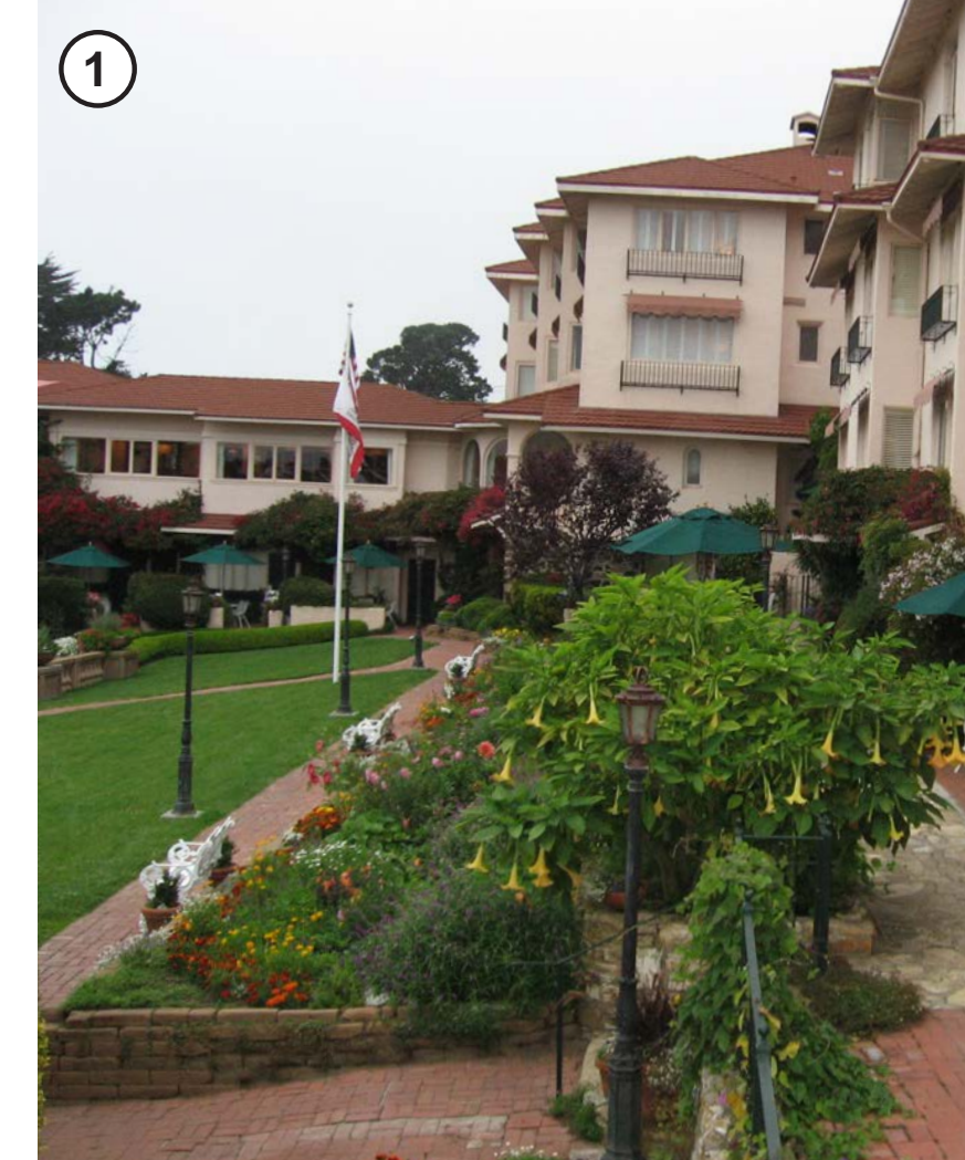
3-story apartments facing gardens
