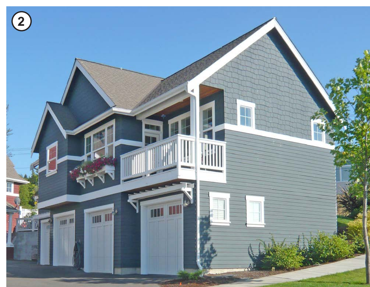
2-story carriage house
