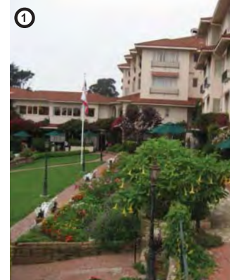
3-story apartments facing gardens
