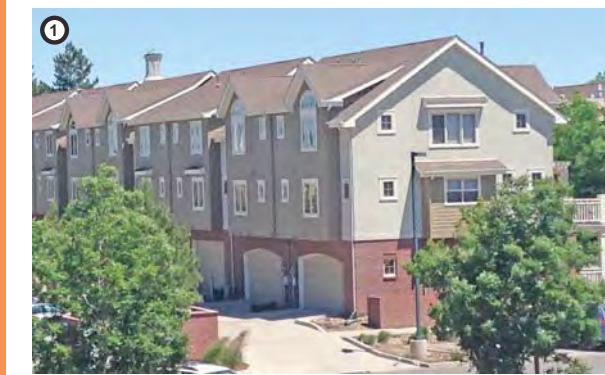
3-story flats with lily-accessed parking in garages
