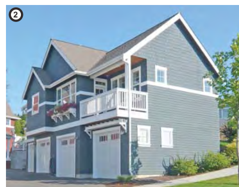
2-story carriage house
