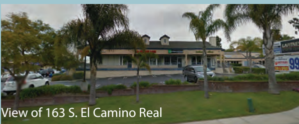
Northbound view of El Camino Real
