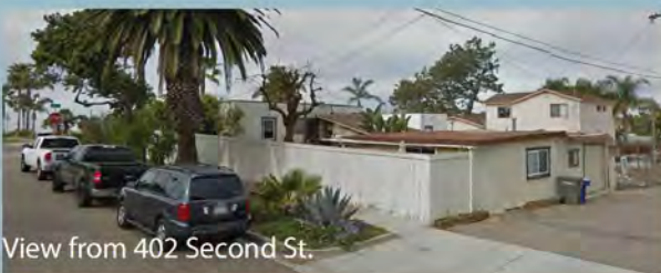
View from Second St./C St. intersection
