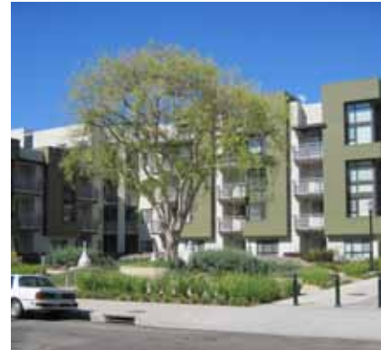
An external courtyard facing a street enhances the public realm while serving residents.
