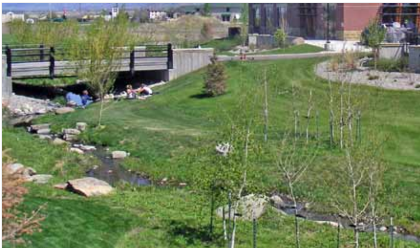
Where on-site stormwater detainage is required, locate landscaping in the path of or surrounding the stormwater swales/basins.
