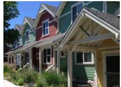
Larger, new development should vary the facades to appear to be smaller, individual structures.
