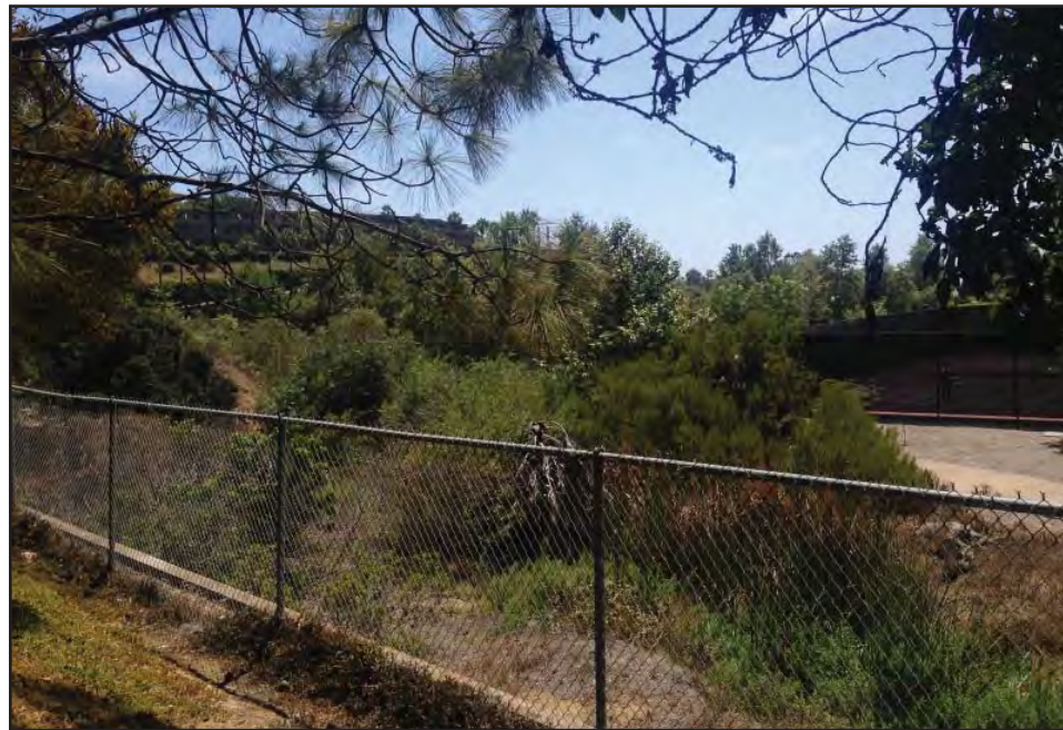
PHOTOGRAPH 88 OE-2 Housing Site
