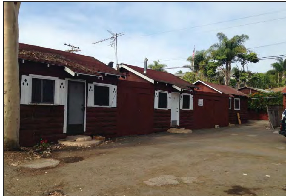
PHOTOGRAPH 11 ALT-2 Housing Site
