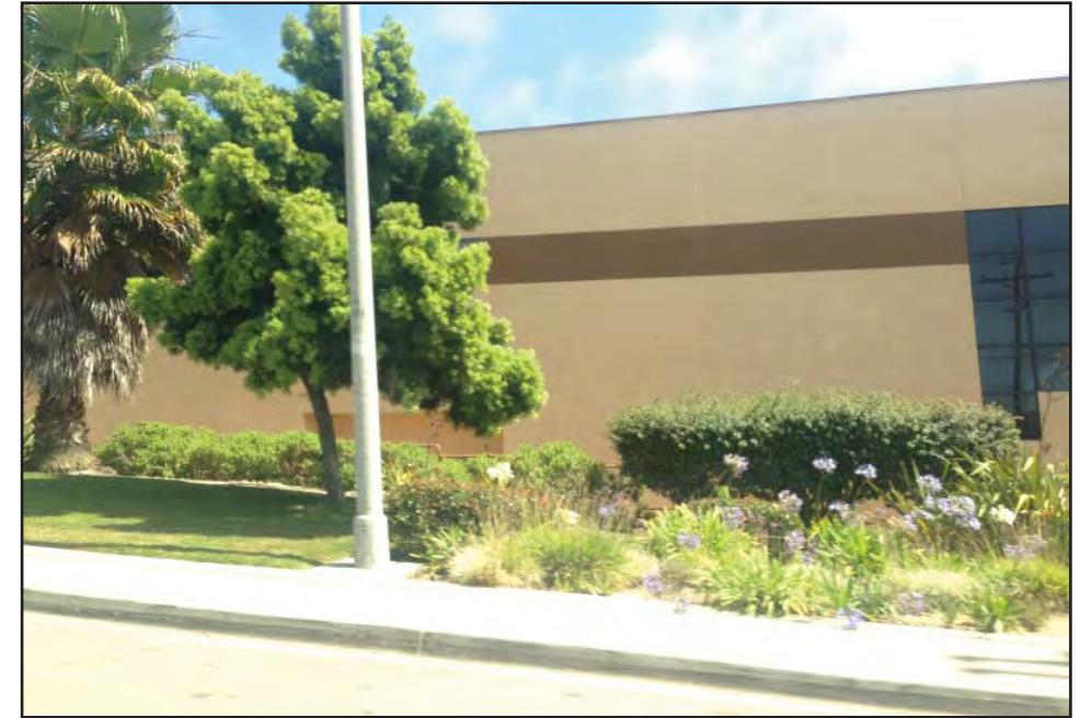
PHOTOGRAPH 111 C-2 Housing Sites
