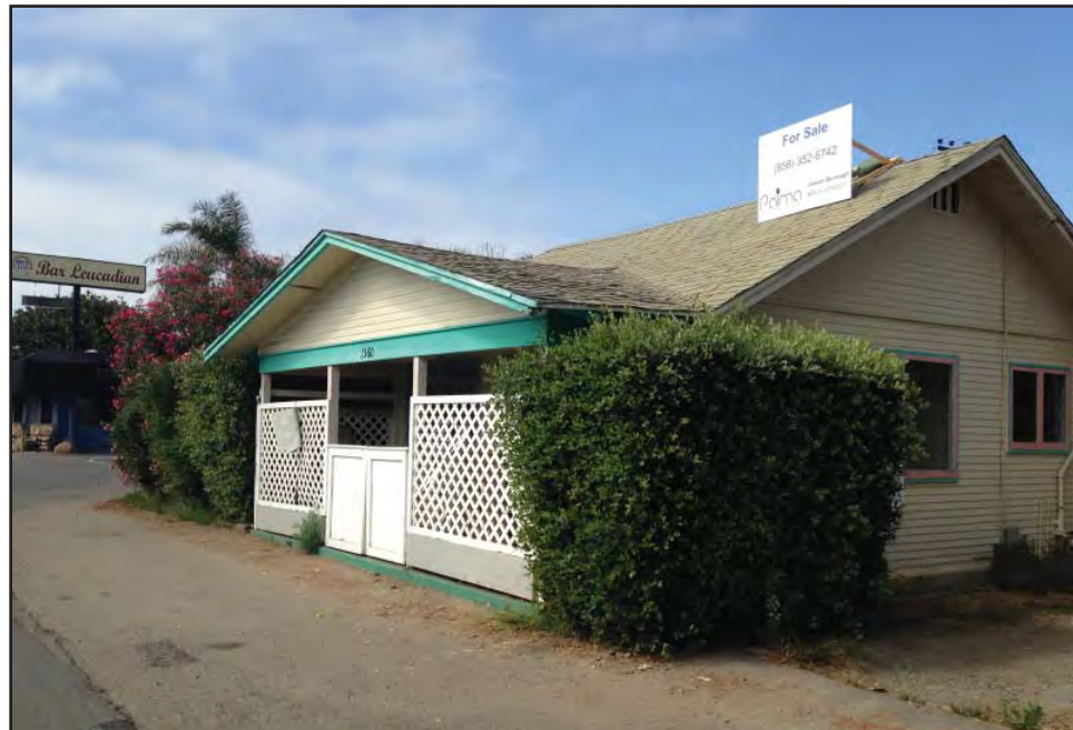
PHOTOGRAPH 16 ALT-2 and L-1 Housing Sites
