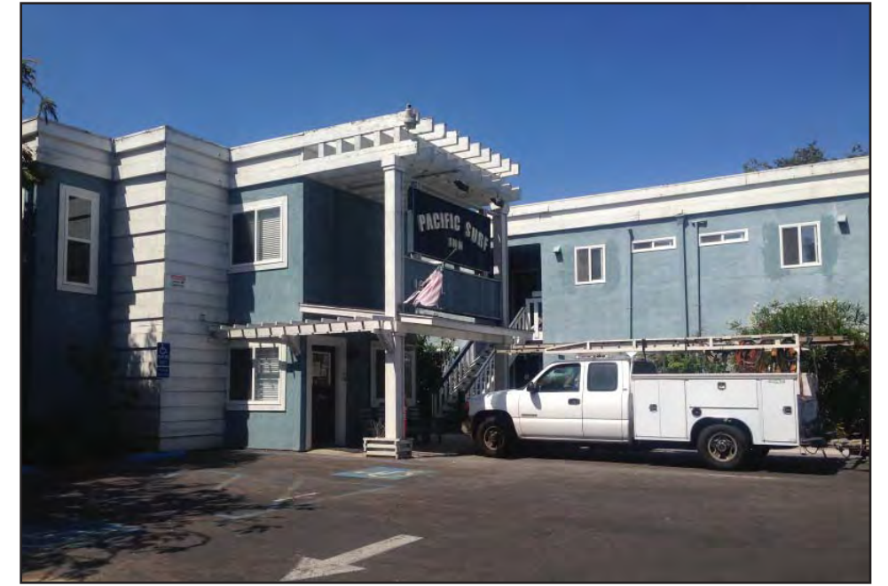
PHOTOGRAPH 33 ALT-2 and L-2 Housing Sites
