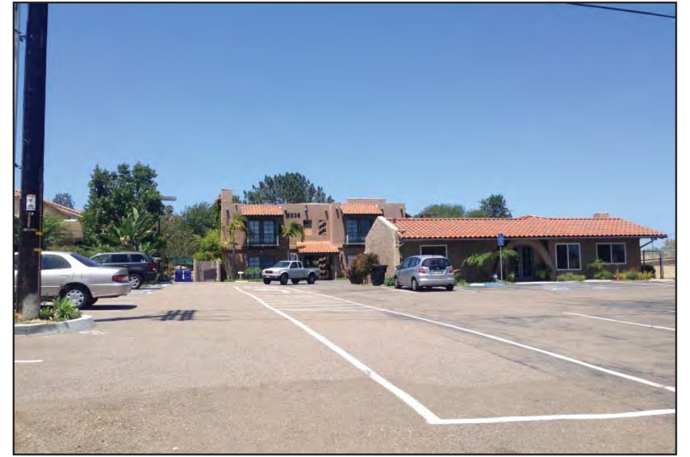
PHOTOGRAPH 73 O-3 Housing Site
