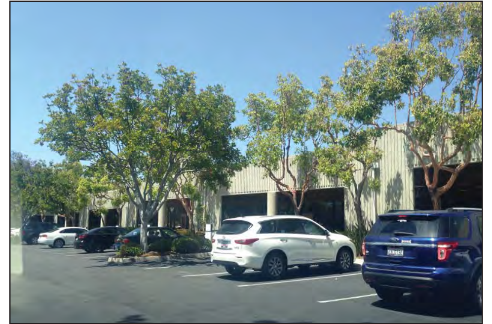
PHOTOGRAPH 83 OE-8 Housing Site
