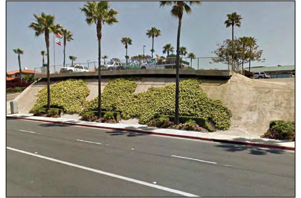
PHOTOGRAPH 89 OE-4 Housing Site
