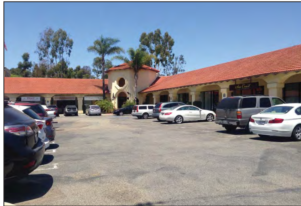
PHOTOGRAPH 75 O-3 Housing Site
