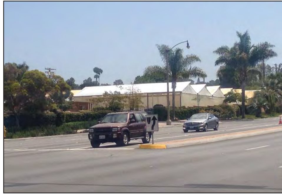
PHOTOGRAPH 42 L-6 Housing Site
