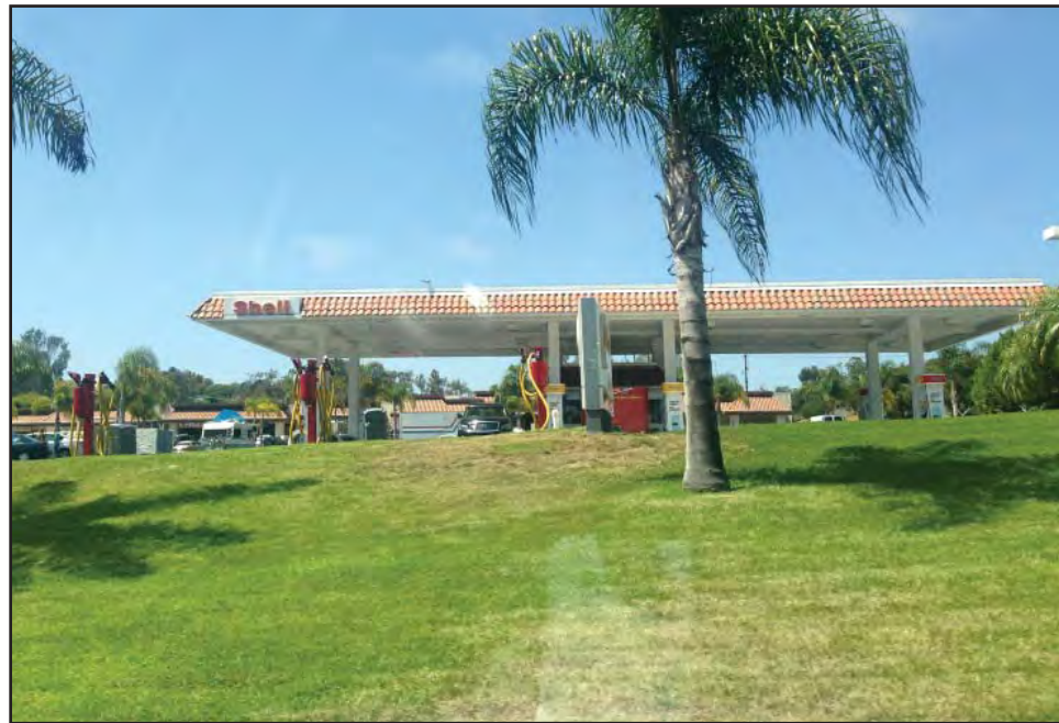
PHOTOGRAPH 87 OE-2 Housing Site
