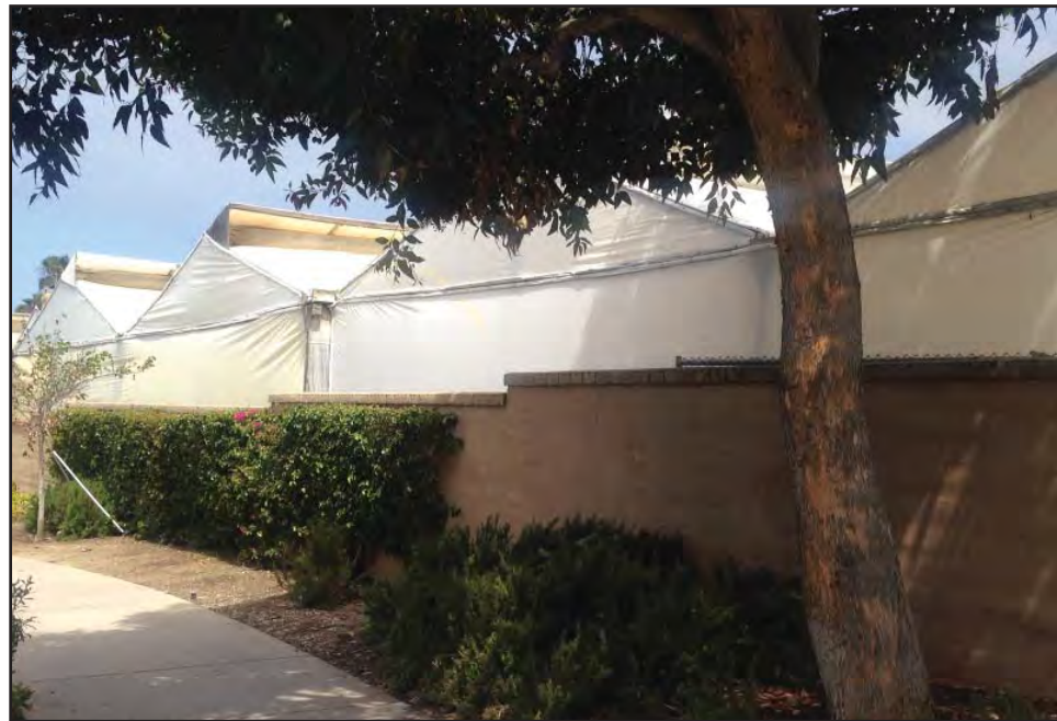
PHOTOGRAPH 44 L-6 Housing Site
