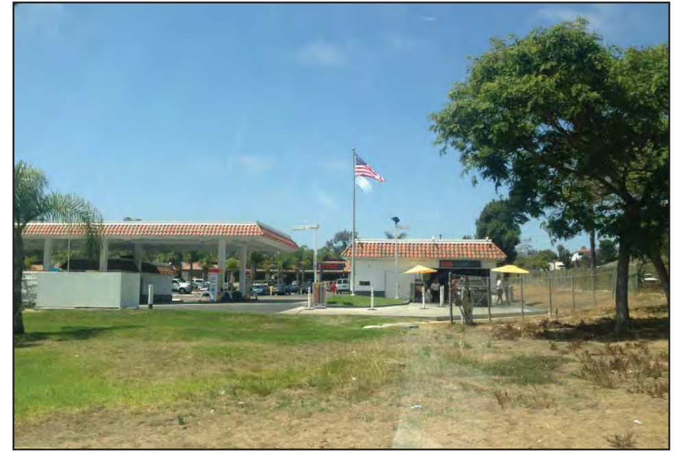
PHOTOGRAPH 86 OE-2 Housing Site
