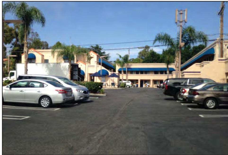
PHOTOGRAPH 22 ALT-2 and L-1 Housing Sites
