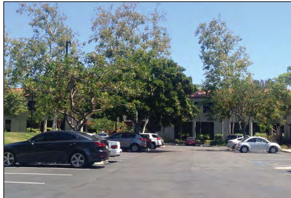
PHOTOGRAPH 82 OE-8 Housing Site
