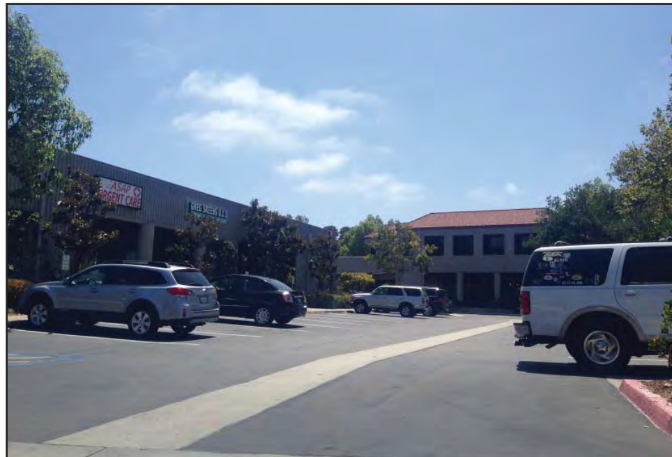
PHOTOGRAPH 81 OE-8 Housing Site
