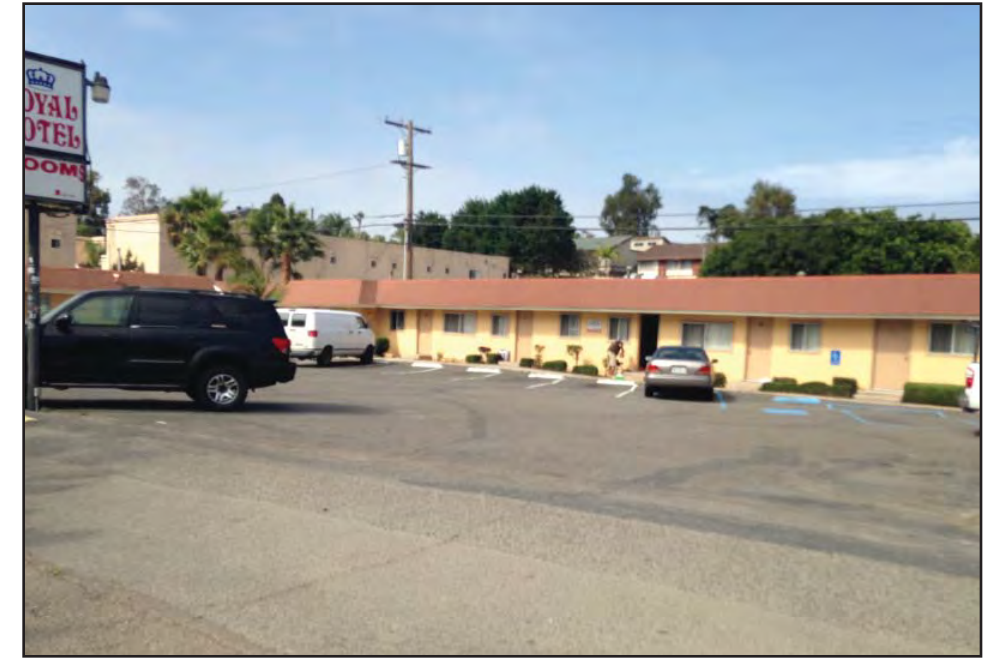
PHOTOGRAPH 21 ALT-2 and L-1 Housing Sites
