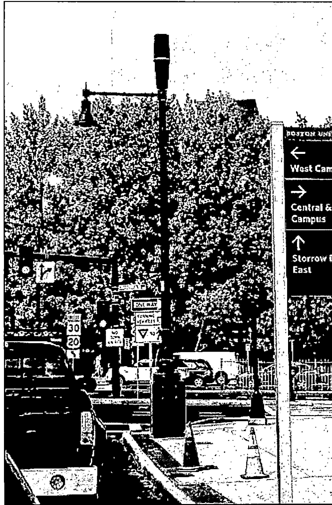
Figure 8: Base-mounted accessory equipment
