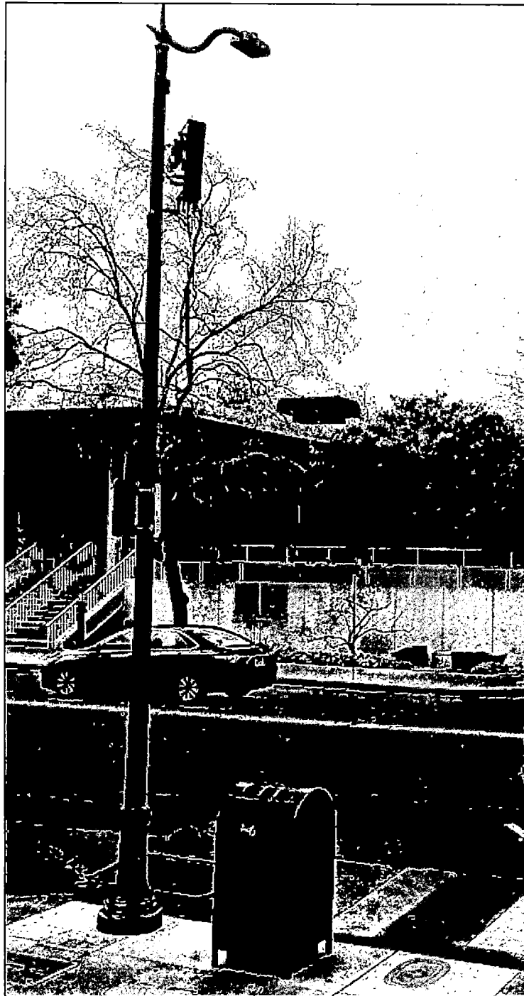
Figure 9: Ground-mounted accessory equipment concealed as a mailbox
