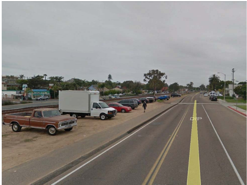
Parking within the NCTD Rail right-of-way along Vulcan Avenue in Leucadia
