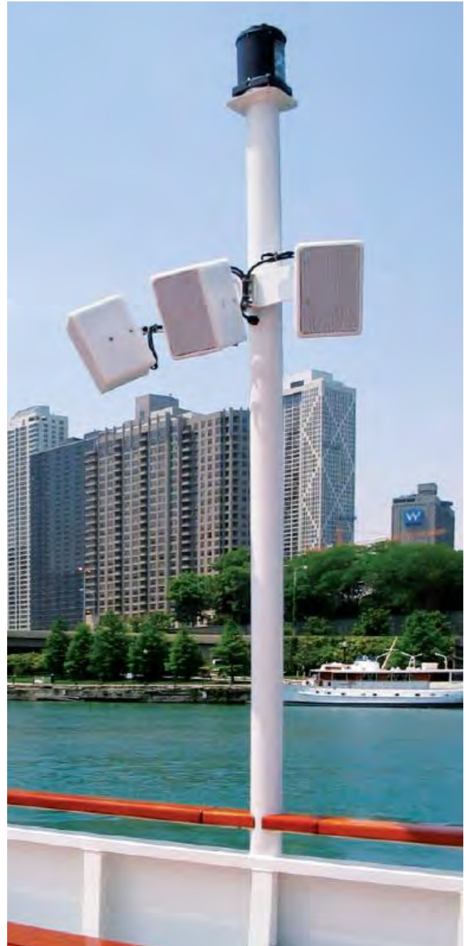
Photo 14—4. Pole-mounted Vernal 15s adjacent to Hong Kong Harbor
