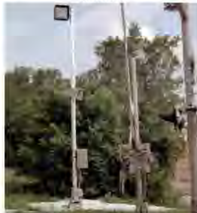
Figure 5. AHS Installation in Mundelein
