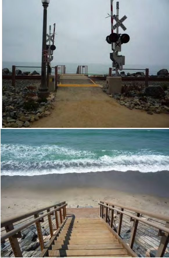
El Portal crossing Beach stairway at El Portal crossing
