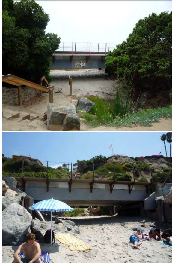
El Portal Grade-Separated crossing
