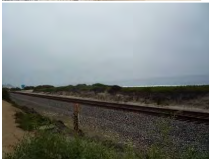
Gap at trail railing and ROW fence
