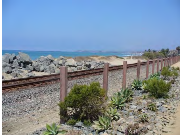
Fencing between North Beach and Dije Court crossings
