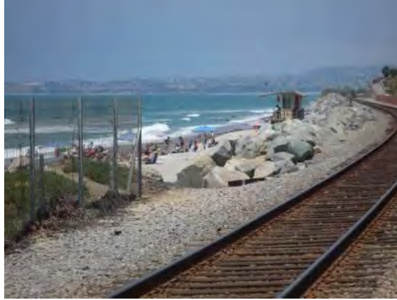
End of fence north of crossing on beach side
