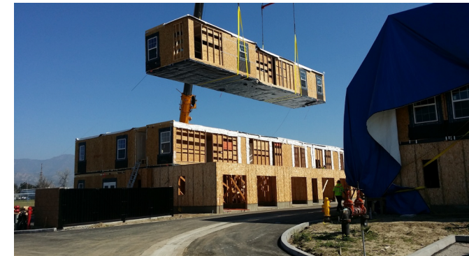
Mixed-use modular construction
