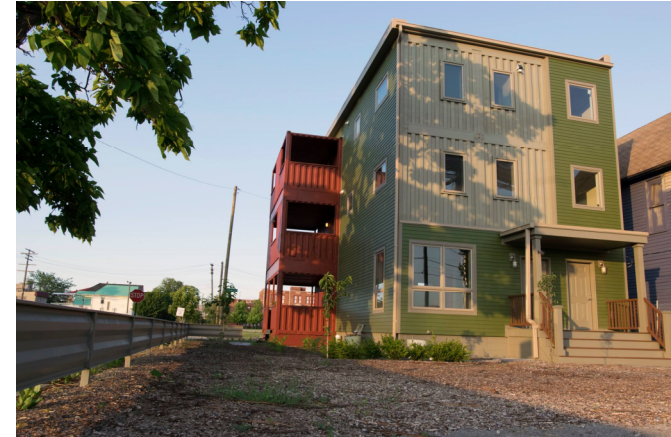
Shipping container construction
