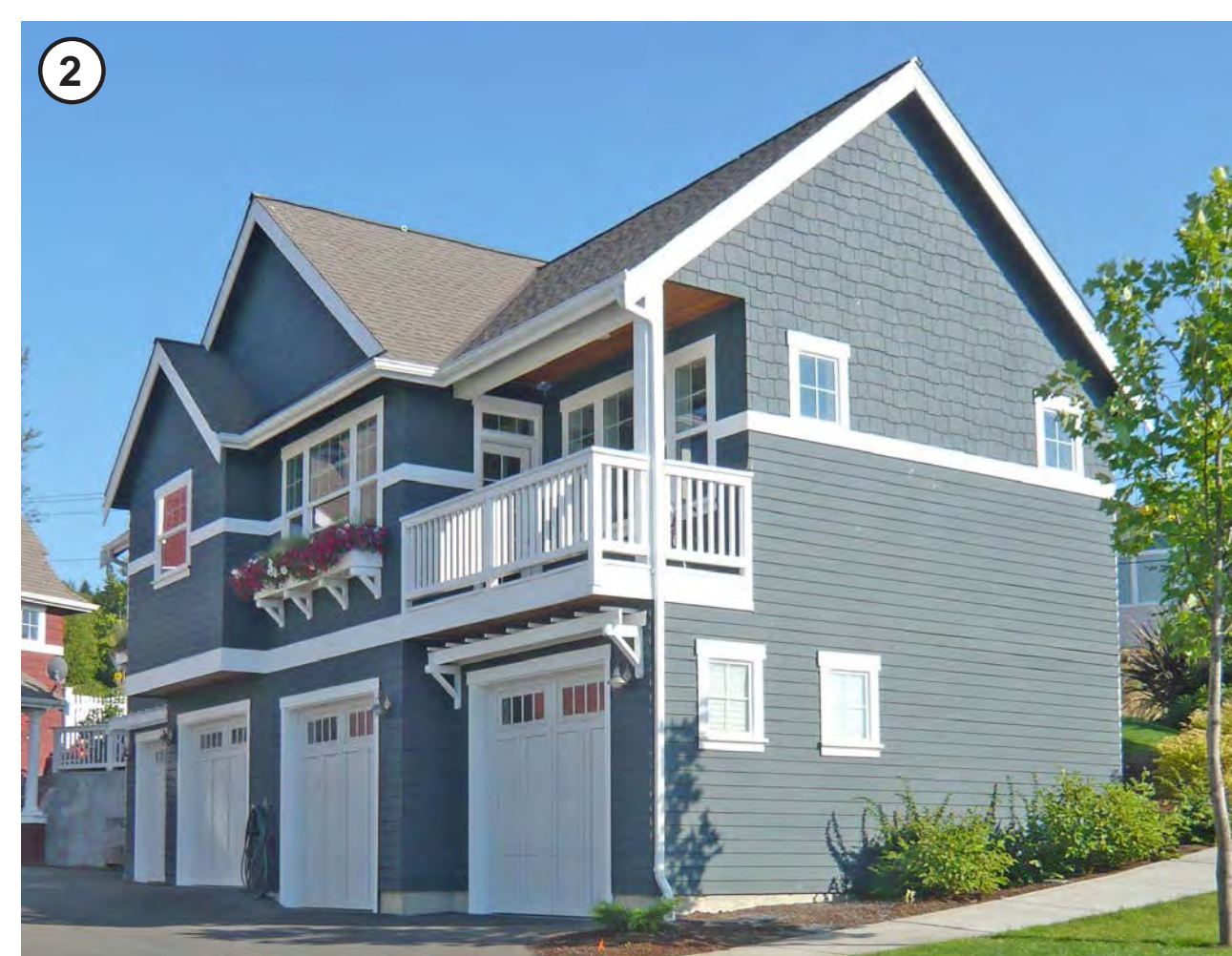
2-story carriage house
