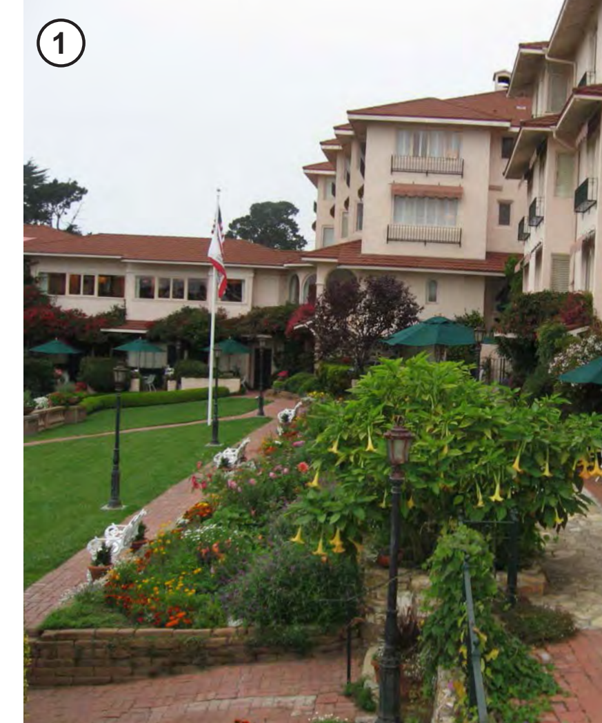
3-story apartments facing gardens
