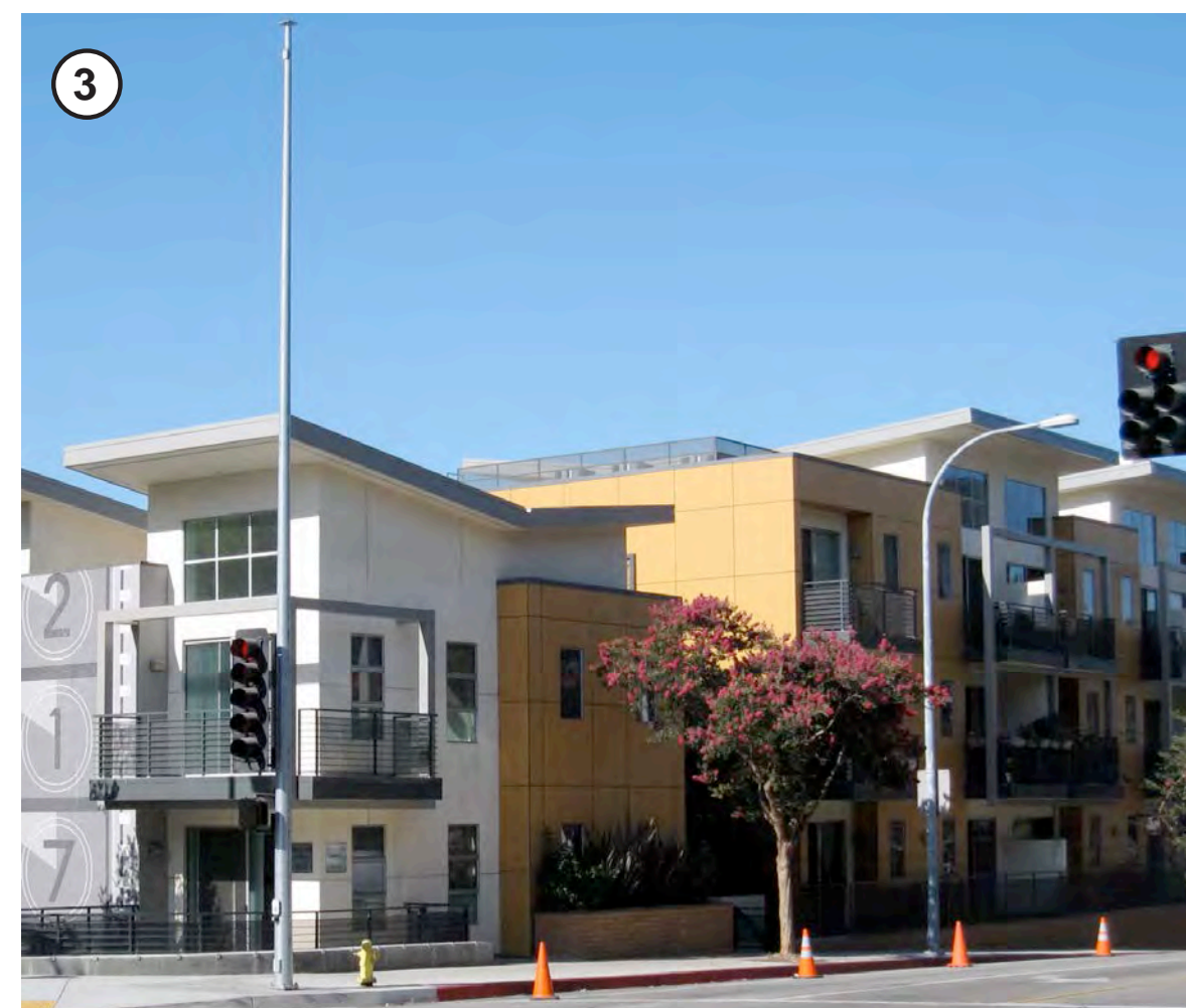
Two and three-story flats
