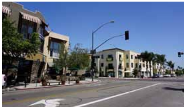
The Kensington Commons project turned a desolate but high-profile corner of Adams Avenue into an oasis of urban living. (Photo by Allard Jansen Architects)
