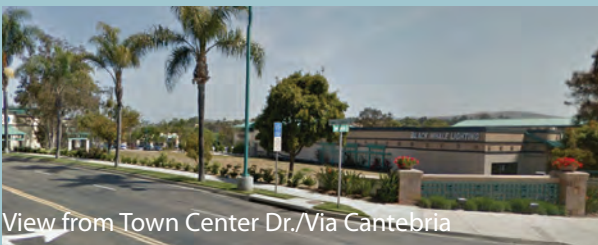
Westbound view from Town Center Dr.
