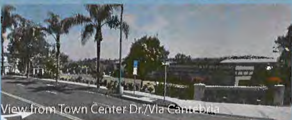
Westbound view from Town Center Dr.
