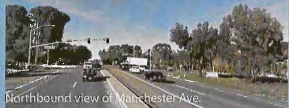
View from El Camino Real/Manchester Ave. Intersection
