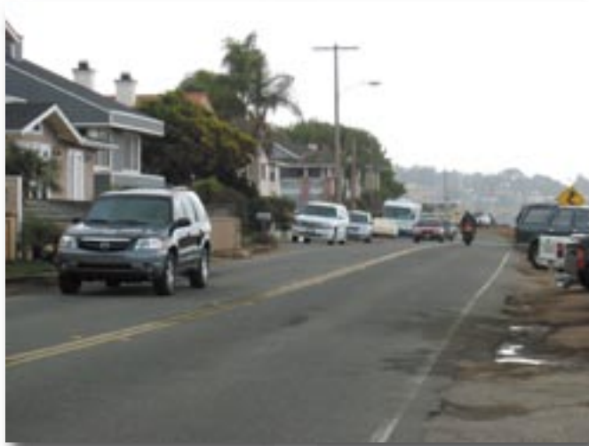
San Elijo Avenue - Crumbling pavement edges correspond with off-street and on-street parking
