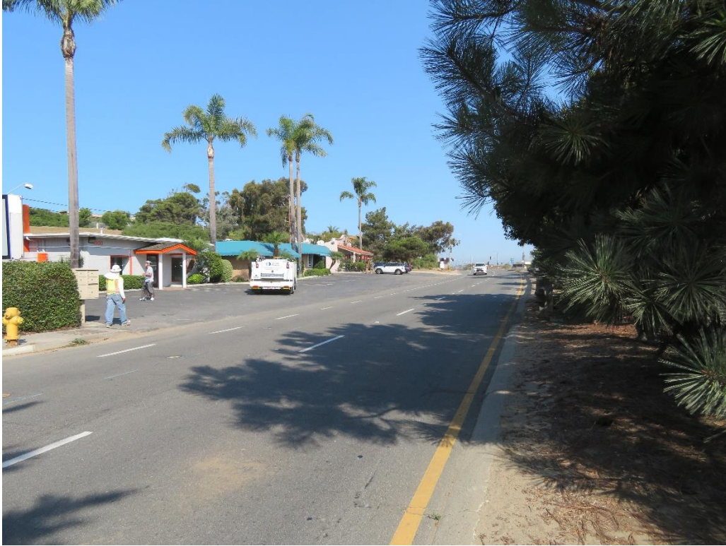
Photograph 7: Photograph of North Coast Highway 101 to the adjoining east of the project site, facing north.
