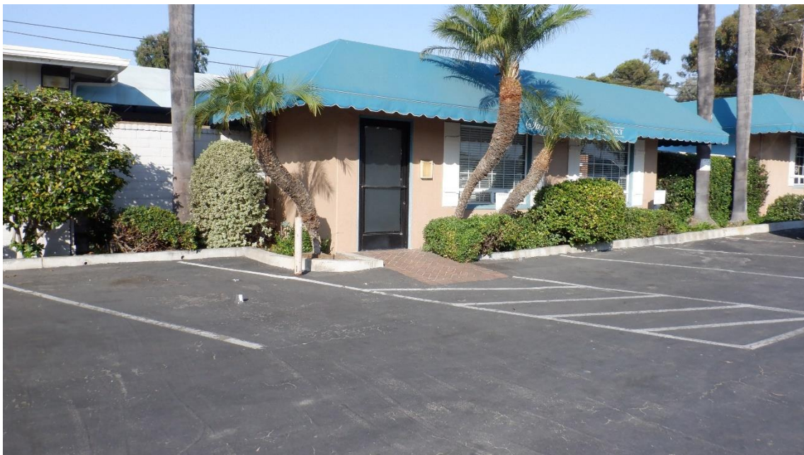
Photo 3. View northwest of Building B at 1900 North Coast Highway 101.
