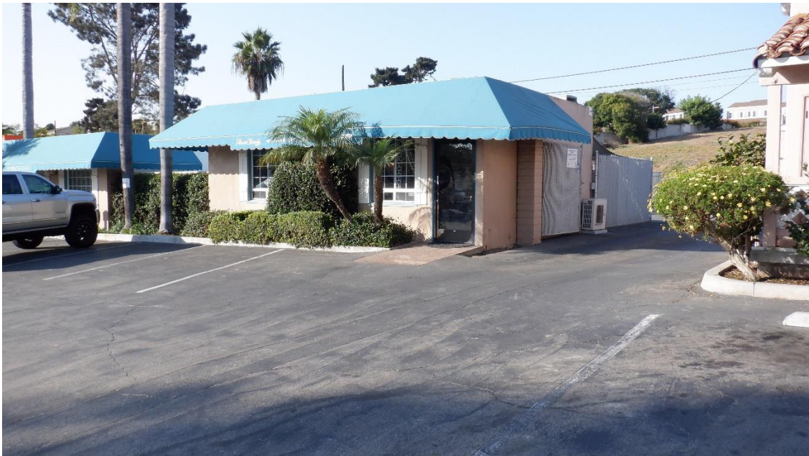
Photo 5. View southwest of Building C at 1900 North Coast Highway 101.
