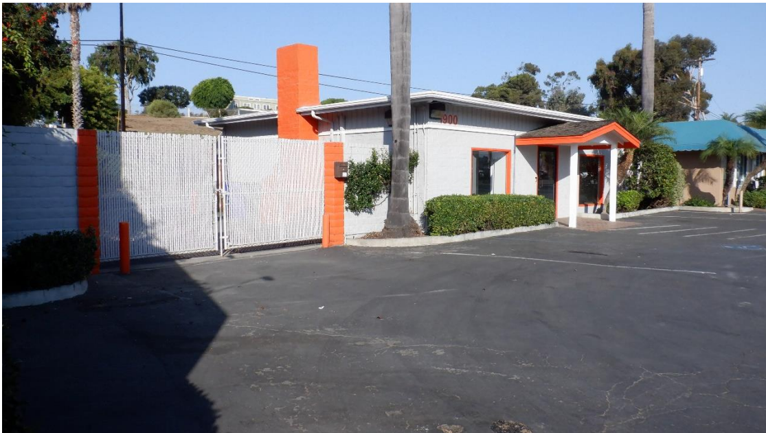
Photo 1. View northwest of Building A at 1900 North Coast Highway 101.
