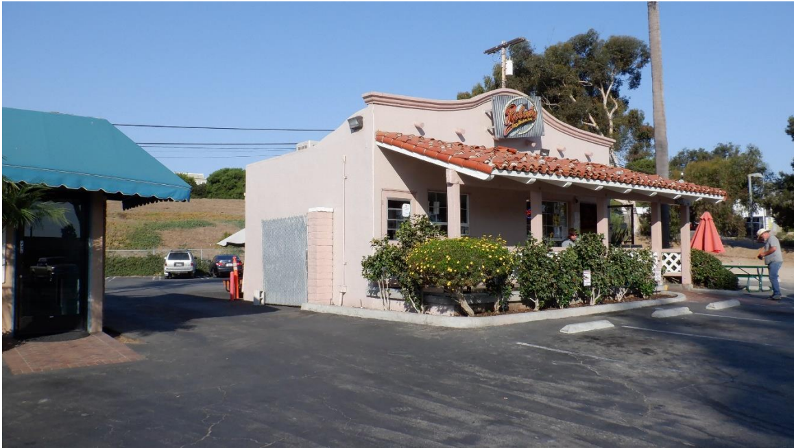
Photo 6. View northwest of Building D at 1900 North Coast Highway 101.
