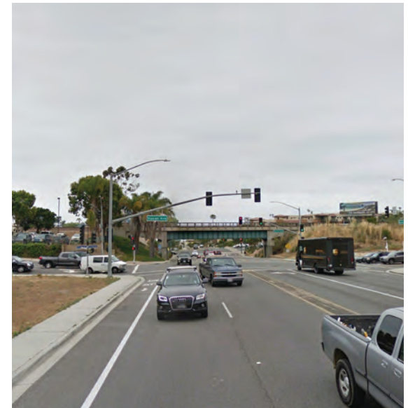
View west down Encinitas Blvd at the Intersection with Vulcan Ave
