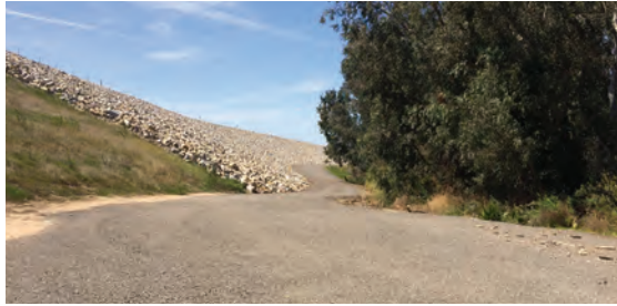
Stabilized/Emulsified Decomposed Granite
