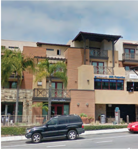
Commercial Uses Along Coast Highway 101
