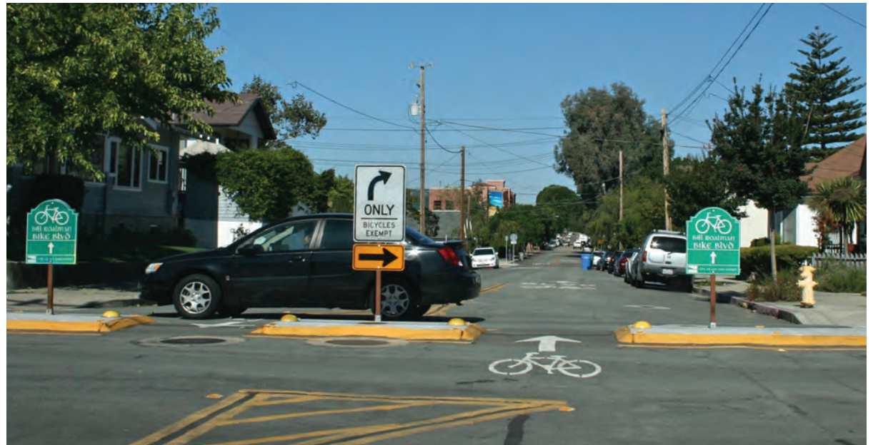
Example of Bicycle Boulevard Vehicle Diverter
