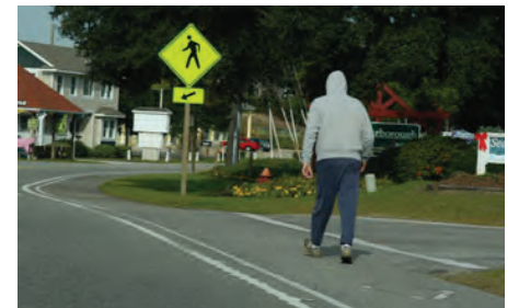
Type 3 Road Edge Enhancement- Where space is tight, stripe at least a 2 foot wide pavement portion
