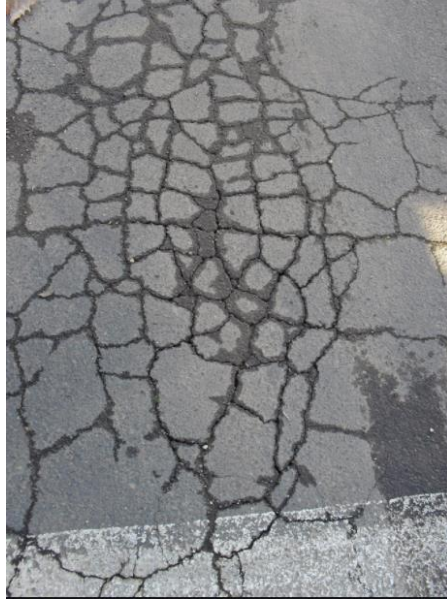
ALLIGATOR CRACKING
