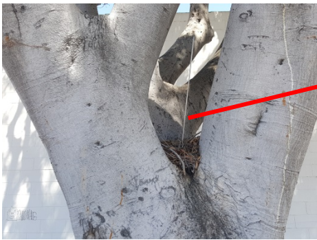
Close-up of cavity
