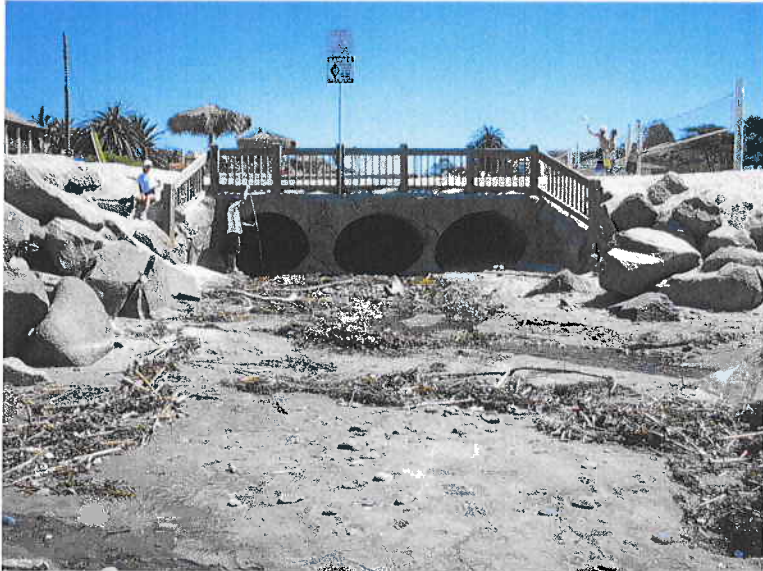
Looking upstream at triple 6'-8" x 5' CMPA
