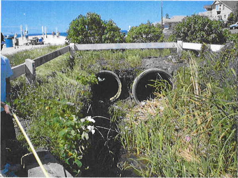
Looking downstream at 60" and 48" RCP
