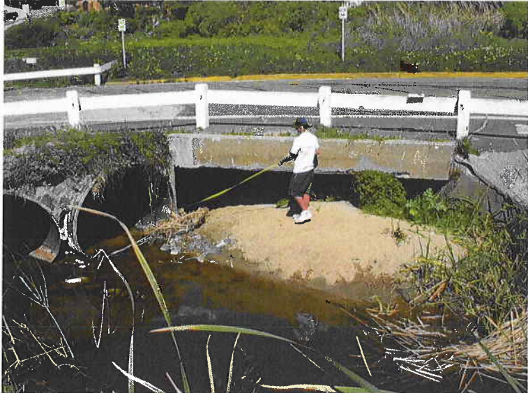
Looking downstream at 10' x 4' RCB that passes under B Street
