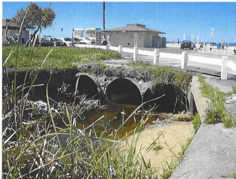
Looking downstream at triple 6'-8" x 5' CMPA
