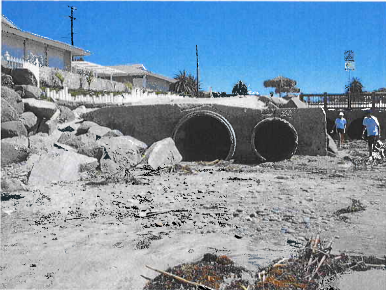
Looking upstream at 60" and 48" RCP
