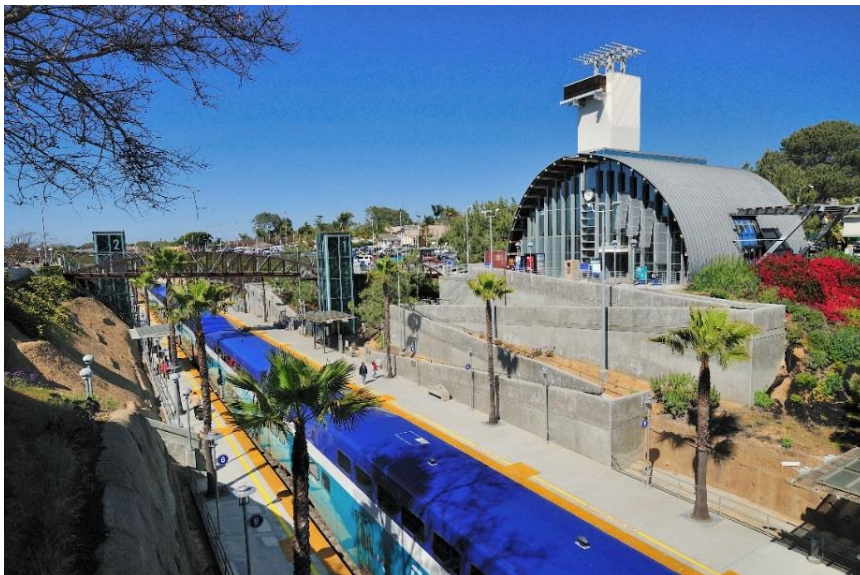
Figure 10: The rail corridor is in a depressed trench in Solana Beach, California, just south of Encinitas. (Caltrans)
