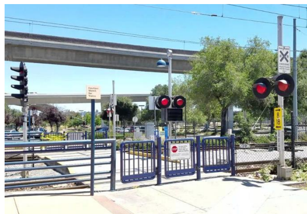
Figure 15: Typical quiet zone supplemental safety measures include (clockwise, from top left): quad gates, quad gates with raised median, pedestrian gates, and a quad gate schematic. (Caltrans; Google)
