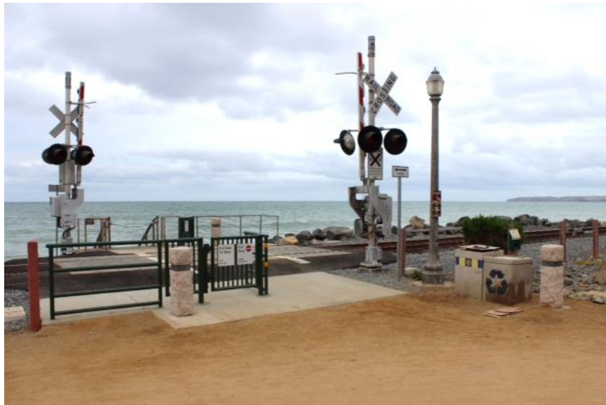
Figure 12: An at-grade pedestrian rail crossing with numerous safety features in San Clemente, California.
