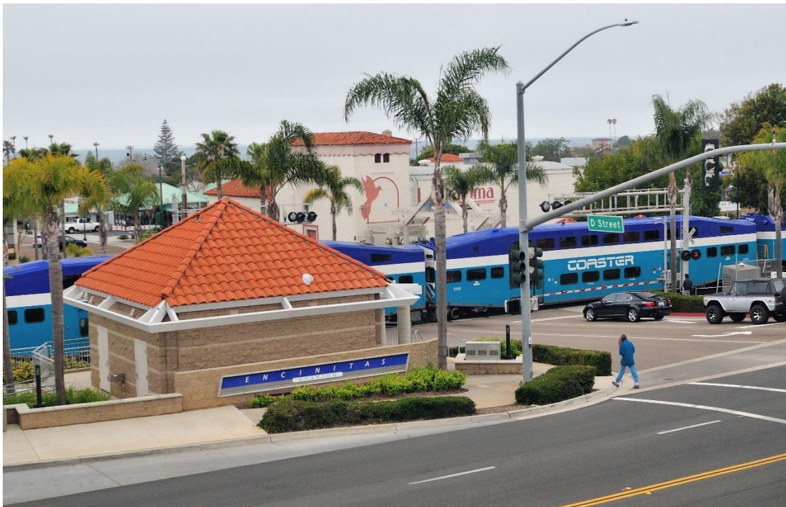
Figure 14: The existing at-grade crossing at D Street will require additional safety improvements to achieve quiet zone status. (Caltrans)
