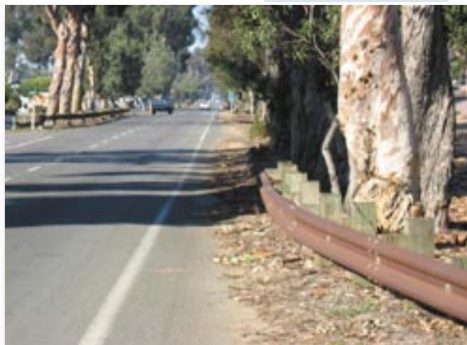
Coast Highway 101 - Guardrails and eucalyptus in close proximity to the traveled way
