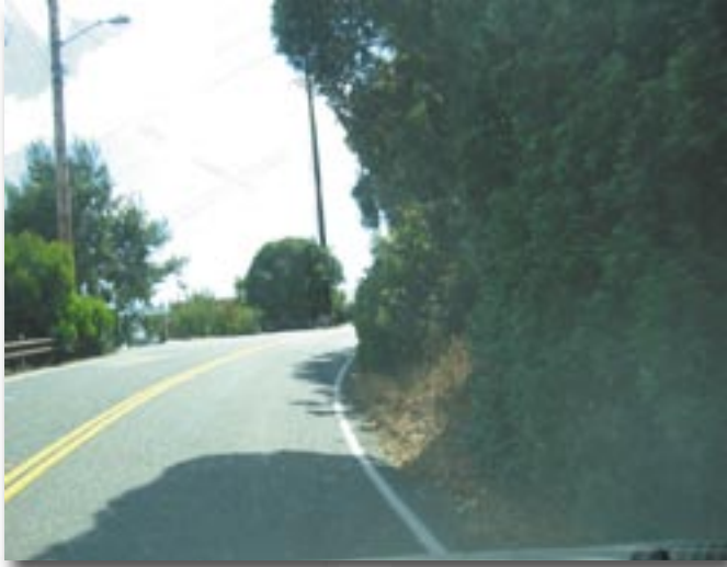
San Elijo Avenue - Narrow roadway with tight curve radii and limited sight distances
