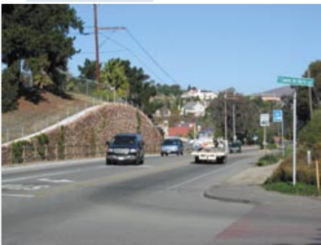
Rancho Santa Fe Road at El Camino del Norte - Retaining wall to accommodate Class 2 bike lane
