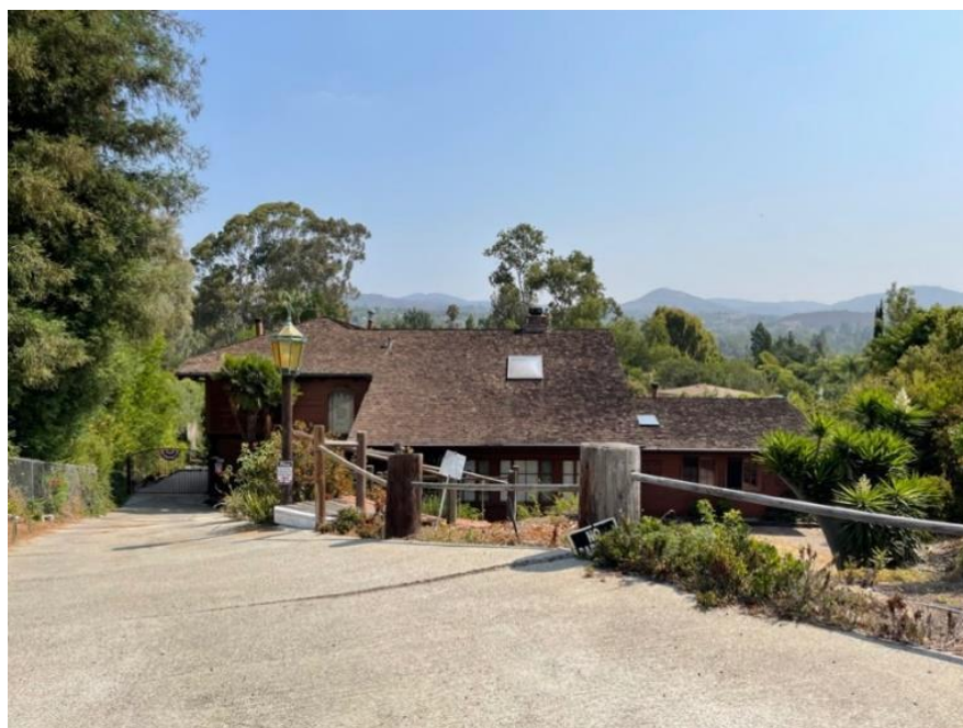
Figure 2: Combustible construction surrounded by highly combustible vegetation
