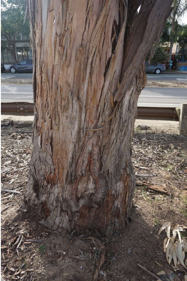
View of wounds on trunk of Tree 20506
