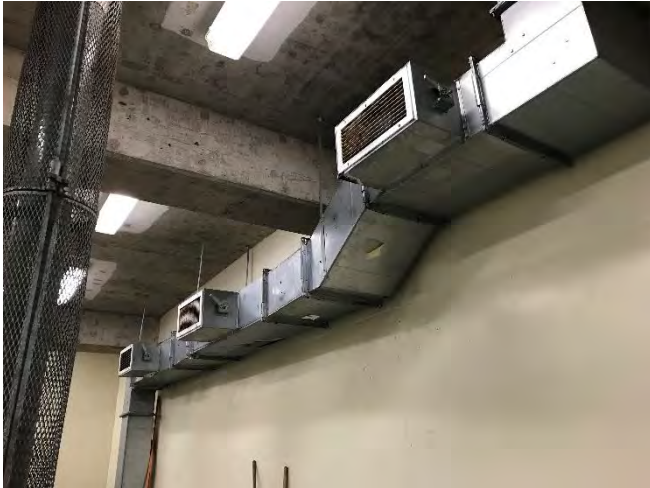
Figure 2.12: Existing Air Supply Ducting and Vents on 2 nd Floor
