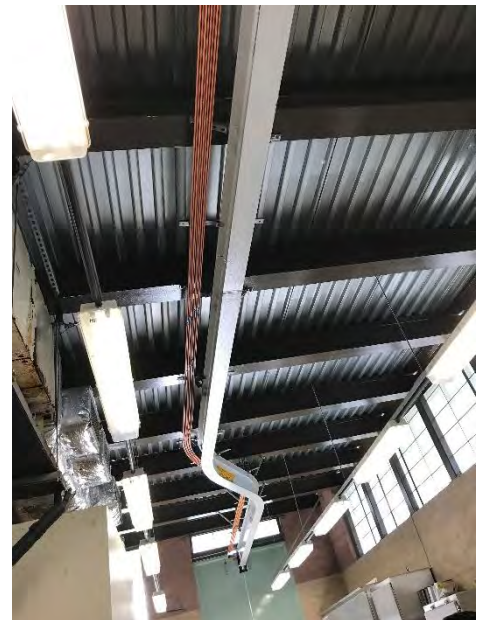
Figure 2.9: Existing 3 rd Floor Monorail Beam Alignment
