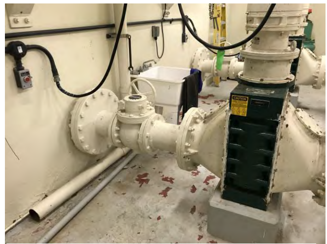
Figure 2.5: Existing Pump Suction Piping and Inline Sewage Grinder View #2
