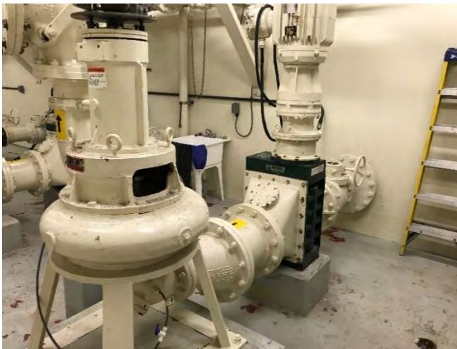
Figure 2.4: Existing Pump Suction Piping and Inline Sewage Grinder View #1
