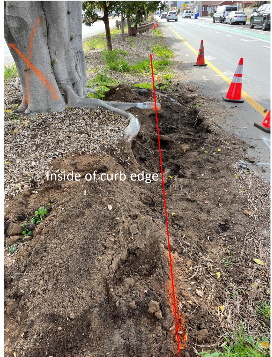
25735E Tree: Detail view of root excavation down to approx. 6 inches below finished grade
