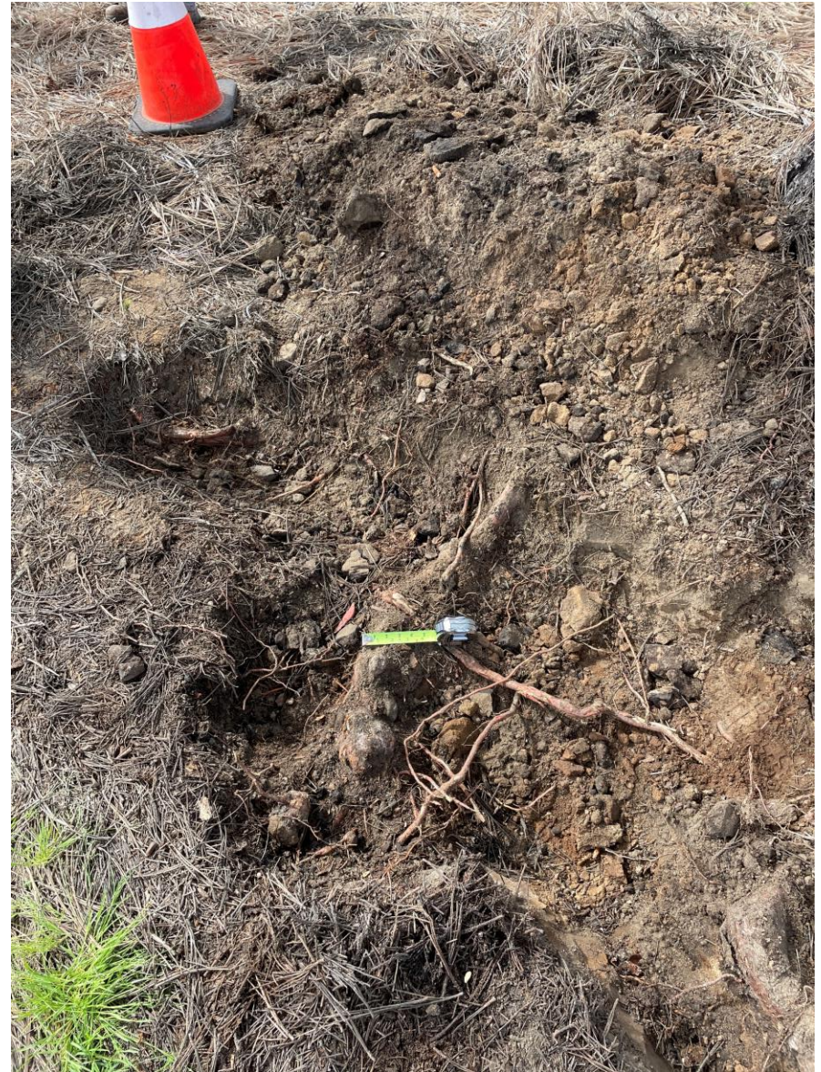
25753E Tree: Detail view of large structural root
