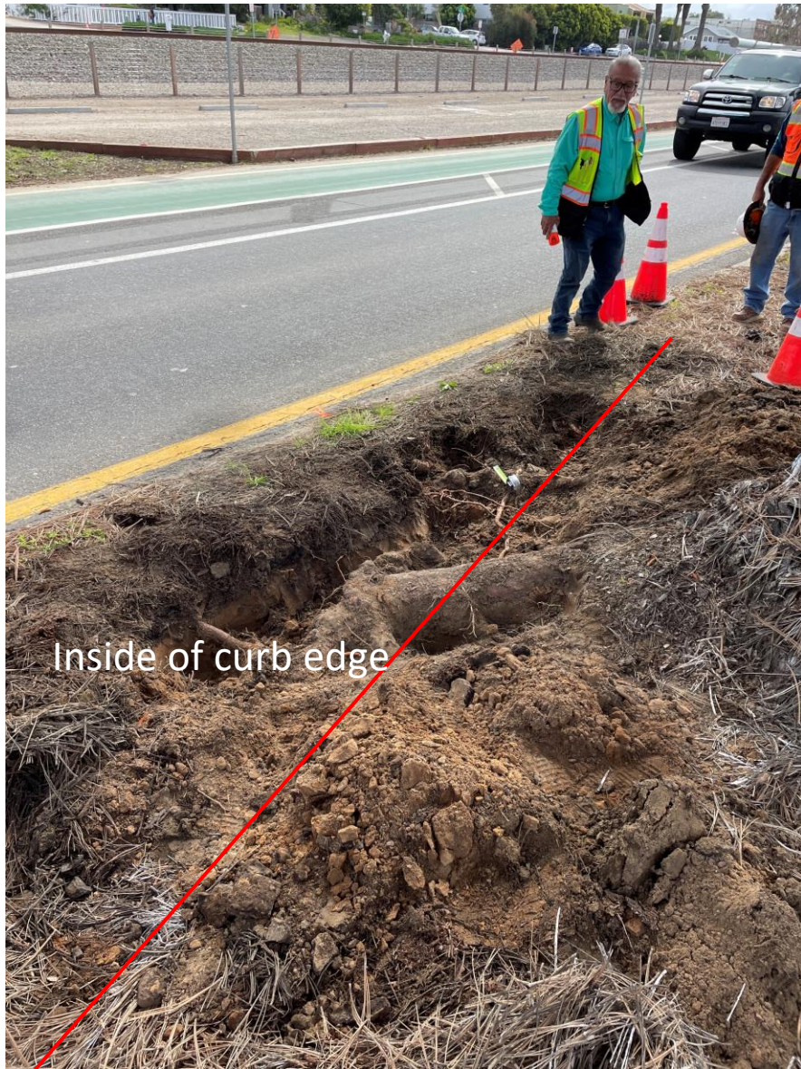
25753ETree : Detail view of root excavation down to 6 inches below finished grade
