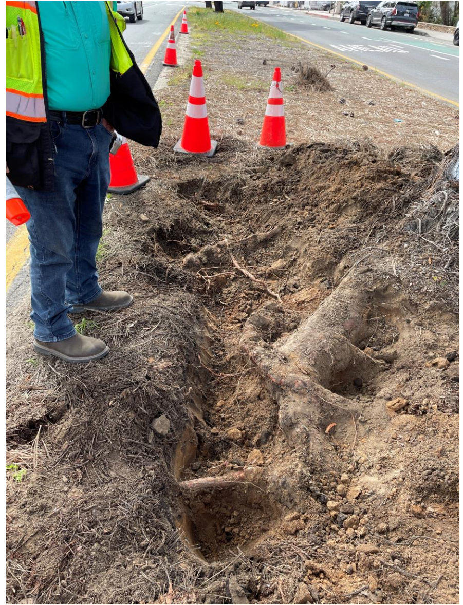
25753E Tree: Detail view of root excavation down to 6 inches below finished grade
