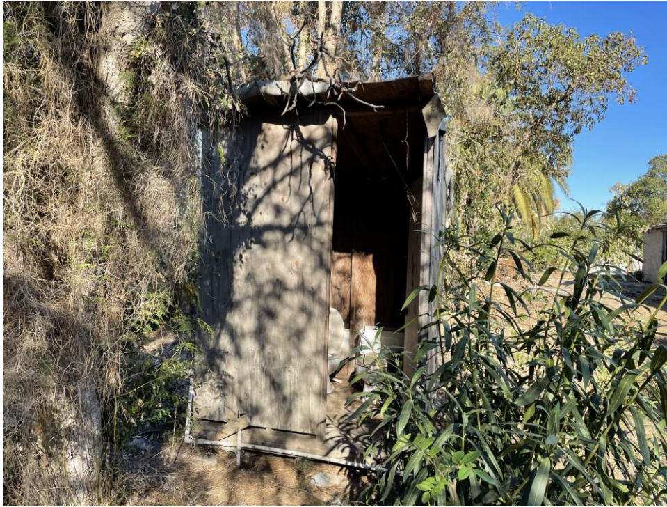
Photograph #13 Outhouse at 1190 Island View Lane.
