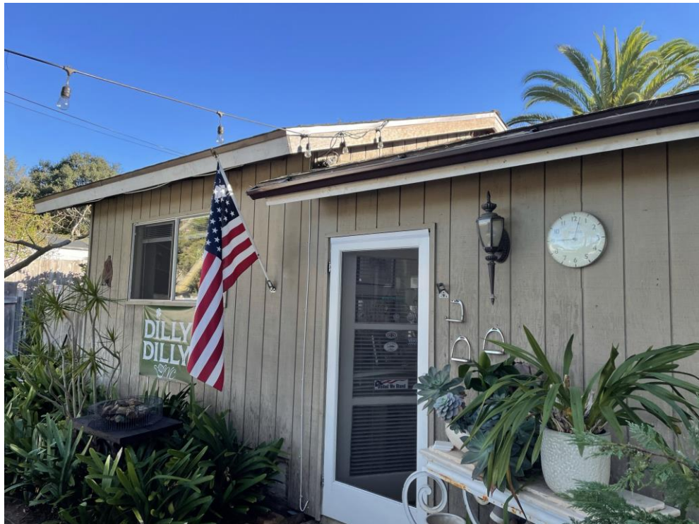
Photograph #2 Single-family residence at 1230A Melba Road.
