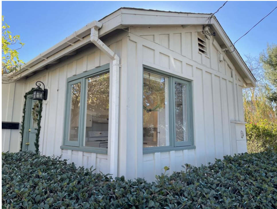
Photograph #3 Single-family residence at 1230B Melba Road.
