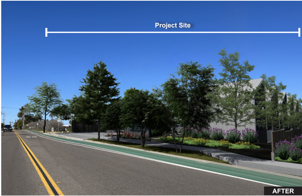
View from westbound La Costa Ave looking west/northwest to Project site.
