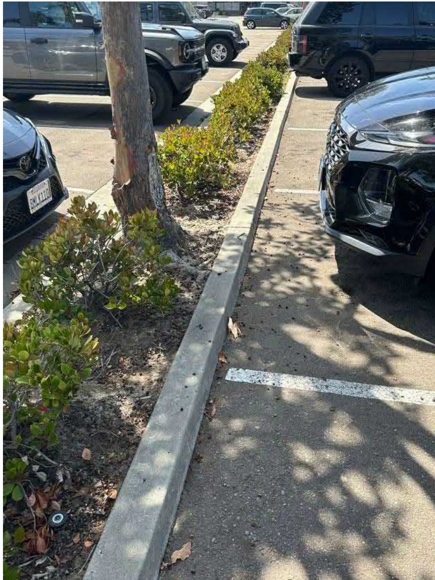
Encinitas Ranch Town Center on El Camino Real Lophostemon confertus – Brisbane box Tree in 3' wide planter damaged by car bumpers which typically extend 2' or more past tires
